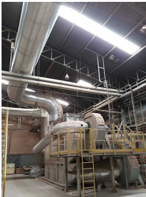
ระบบ Waste Heat Recovery from Kiln's Chimney (Air to Air Heat Exchanger )
