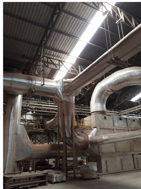
ระบบ Waste Heat Recovery from Kiln's Chimney (Air to Air Heat Exchanger )
