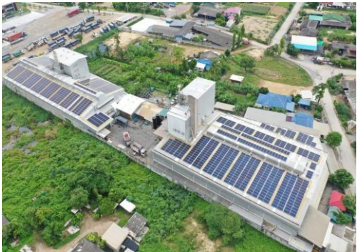
BETAGRO PUBLIC COMPANY LIMITED Solar Roof 430 kWp
