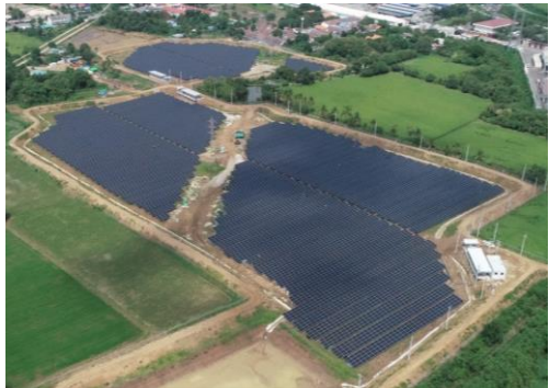
Siam Fiber Cement Group Solar Farm 8,700 kWp
