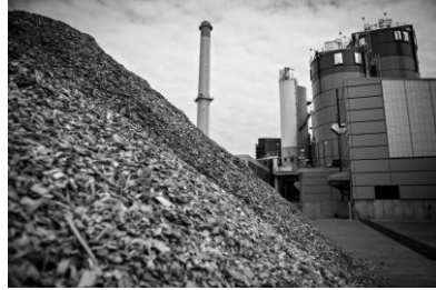
Biomass for Hot Air Generator
