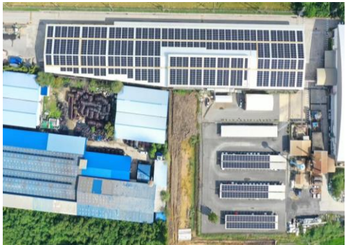
SCG Packaging Company Limited Solar Roof 999.6 kWp
