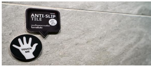
Anti-slip tile with slip-resistance rating 11 or R11
