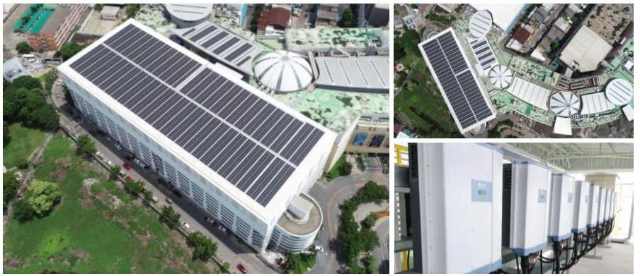
CPN at Central Plaza Rama II 998.8 kWp
