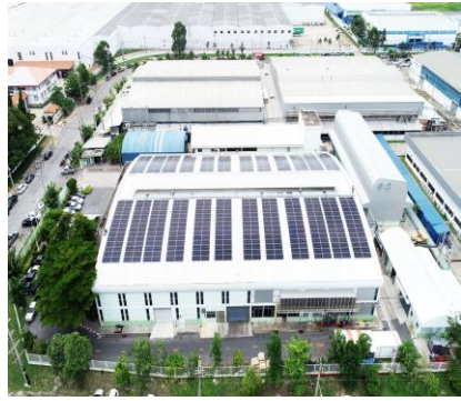
Multibax Public Company Limited 265.44 kWp
