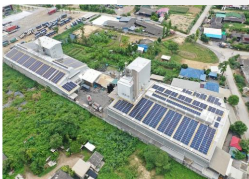
BETAGRO PUBLIC COMPANY LIMITED Solar Roof 430 kWp
