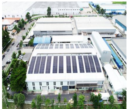
Multibax Public Company Limited 265.44 kWp
