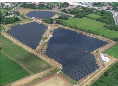
Siam Fiber Cement Group Solar Farm 8,700 kWp
