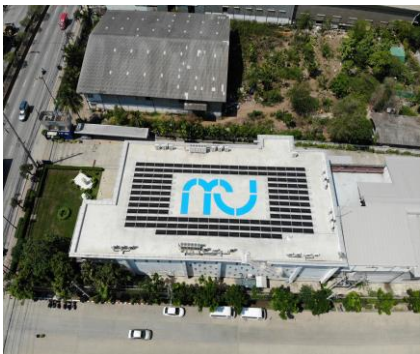
M.J. Bangkok Valve & Fitting Co., Ltd 56 KwP
