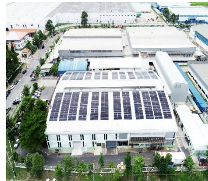
Multibax Public Company Limited 265.44 kWp
